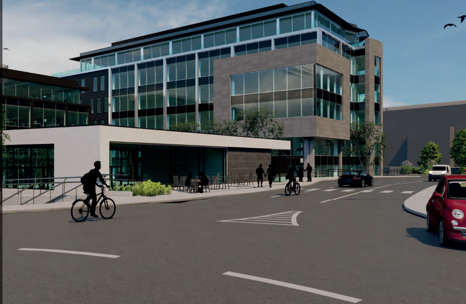
Indicative external south-west day view
